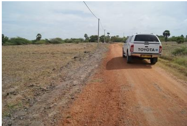
Pic: Road and paddy field remain at the same elevation, leading to frequent flooding.
