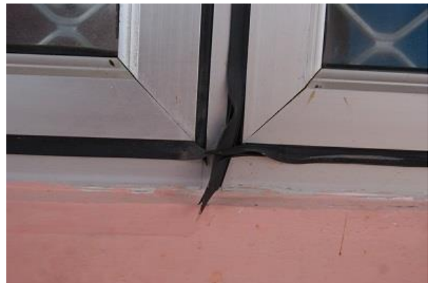
Pic: Some unfinished works.
