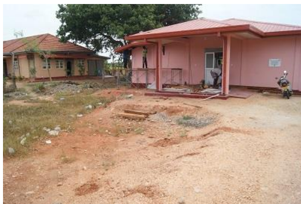
Pic: Front area where backfilling is needed
